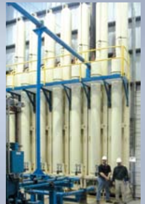
Large accumulator system for wood presses
