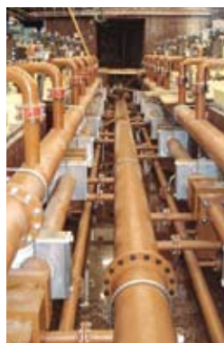
Deep drawing, metal forming, and base-forming presses for pressure equipment production: Offline filter circuit 1,000 l/min, pressure 6 bar Commissioning on site including assembly and installation
