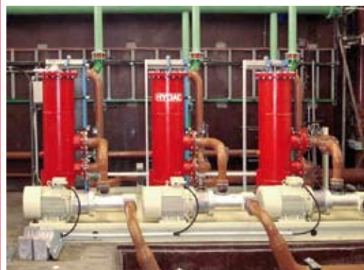
Deep drawing, metal forming, and base-forming presses for pressure equipment production: Offline filter circuit 1,000 l/min, pressure 6 bar Commissioning on site including assembly and installation
